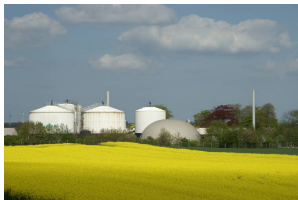
Figure 6.1. Biogas plants contribute to a better utilization of nutrients in the agriculture. Photo courtesy of Torkild Birkmose, DAAS
