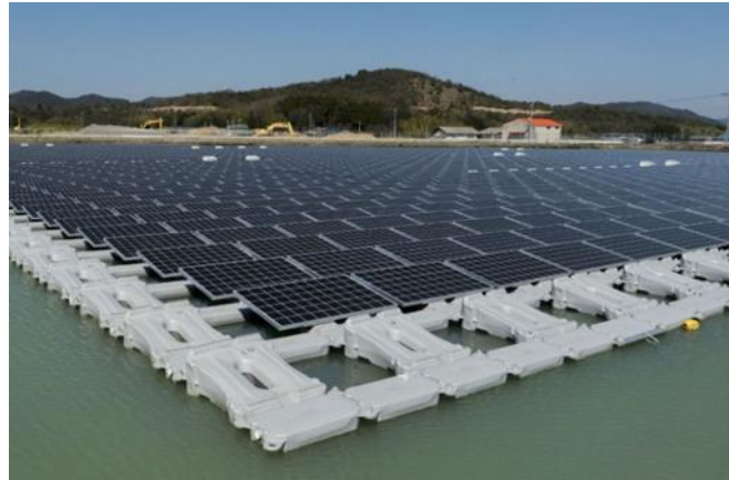
Figure 12. Floating structure from Kyocera for a 13.7 MW FSPV plant [69,70].
