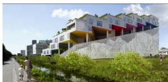
B.I.G. MTH – Boliger, under construction, Ørestaden. Rendering: B.I.G.
