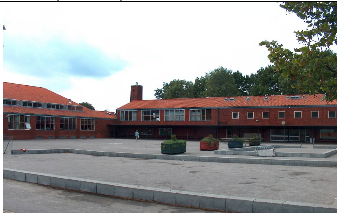
Stengård primary and lower secondary school, Gladsaxe Contractor: Gladsaxe Municipality.
