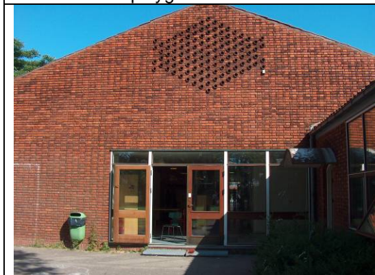
Exit from one of the corridors.
