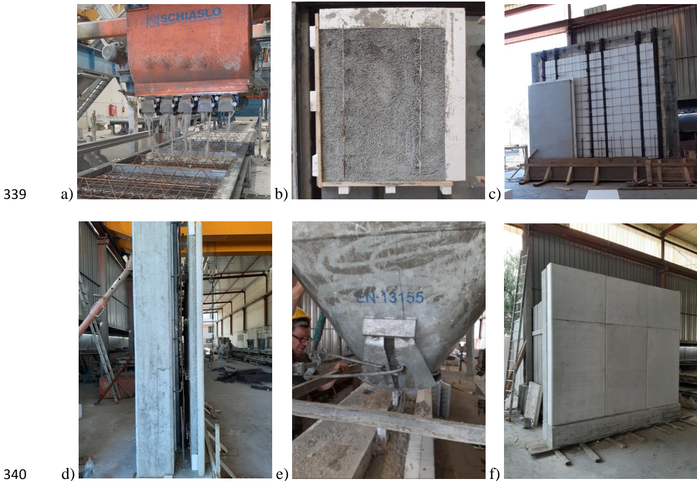
Figure 8 – Construction phases and application of the IPCS prototype: a) constitution of the panel with an industrial process; b) finished IPCS; c) infilled frame with application of one panel; d) lateral detail of the system; e) casting of lightening concrete layer; f) final result of the prototype.
