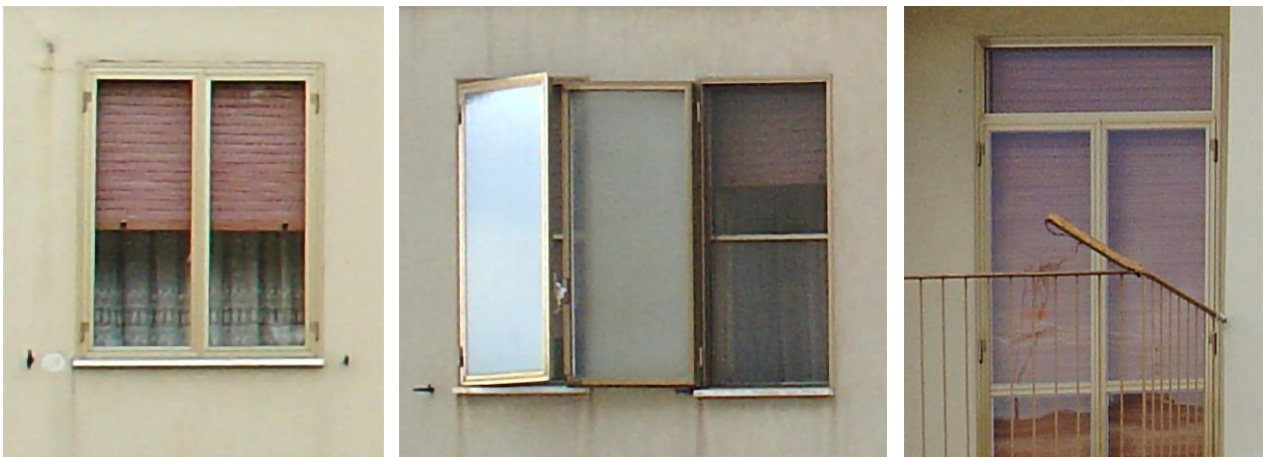
649 Figure 19 – Case study building: survey of the windows.
