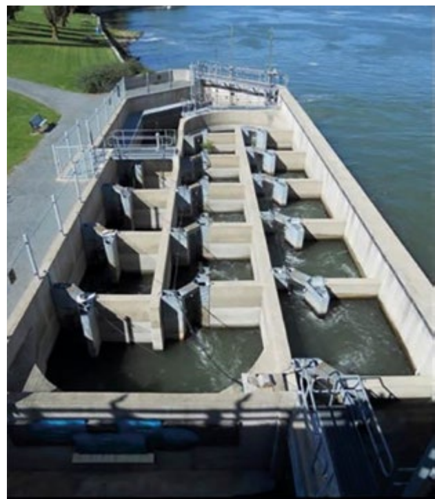
Figure 3. The St. Ours dam on the Richelieu River in Canada has one of the few proven efficient fishways for (lake) sturgeon (Thiem 2013)
