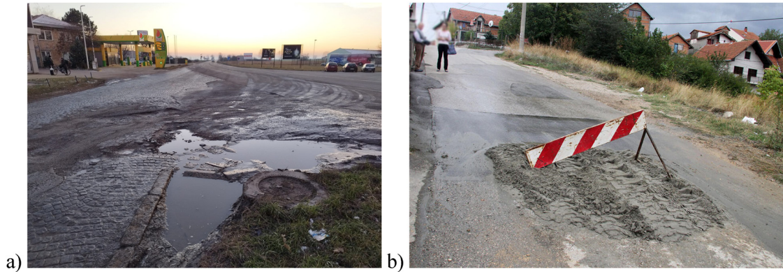
Figure 14: Examples of poor road maintenance in the area of (a) Subotica and (b) Novi Sad. Source: 14a. Authors (12.01.2024), 14b. Dragan Kadić (18.05.2022).
