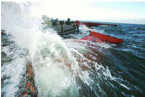
Fig. 2: Waves overtopping the ramp of the Wave Dragon prototype in Nissum Bredning, Northern Denmark.
