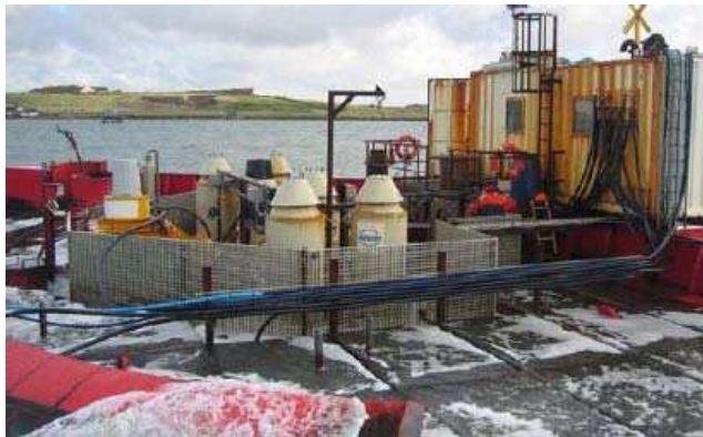
Fig. 12: Trash rack with 5 x 5 cm grid openings enclosing the turbine area.
