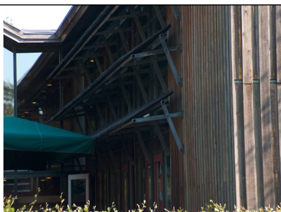
Solar shading over all windows.
