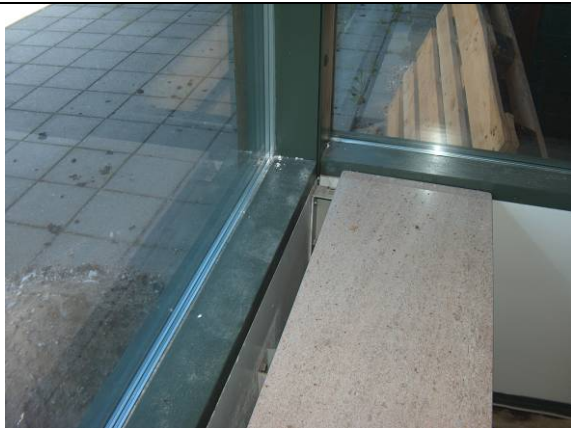
Window wall in sheltered homes.
