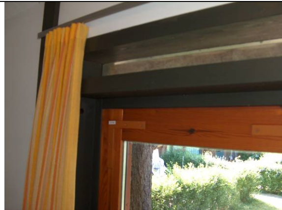
Single glass windows above doors.
