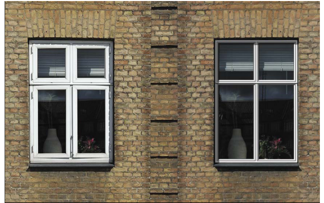
Figure 33. The new GRP window shown to the right alongside a window from the 1980s.
