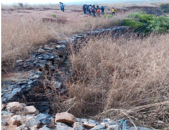
Plate 8. Stone pitching reclamation at Kuru Kuru
