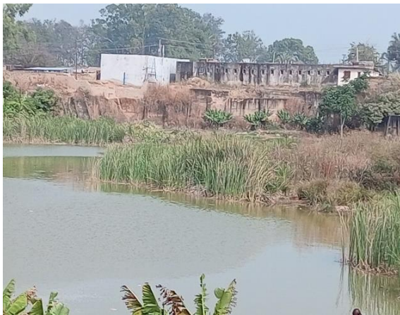
Plate 10. Wall retention constructed at Bukuru, Jos
