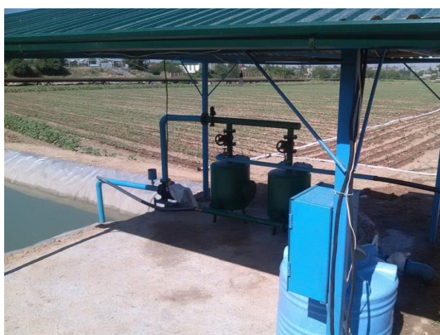
A pool of water storage in drip irrigation
