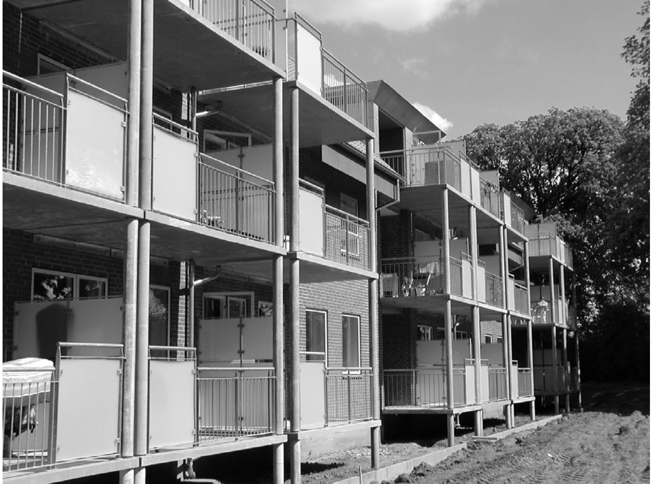
Figure 10 CRC Balcony slabs and columns produced by Hi-Con at Askehaven, Vejle in Denmark.
