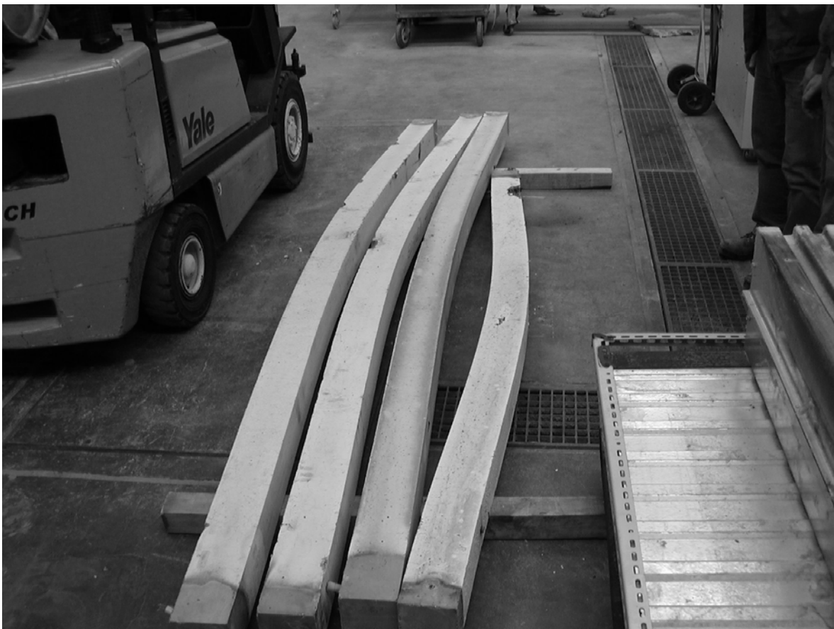
Figure 9 - Some of the columns after fire exposure.
