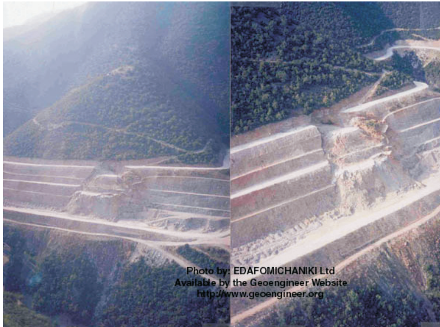
Figure 1.4 Example of a highway slope failure in Greece. ( www.geoengineer.org ).
