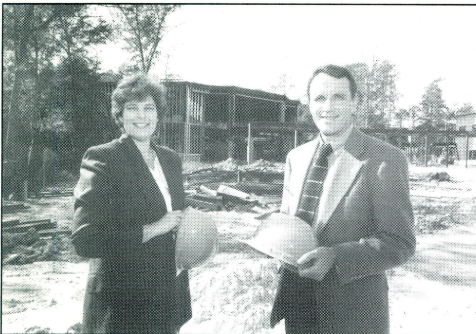
Montgomery College President Bill Law, right, and Mary O'Neil, Vice President of Educational Programs and Resources, inspect the building of the new college, due to open in fall 1995.
