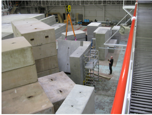
(a) Concrete blocks for bunker walls
