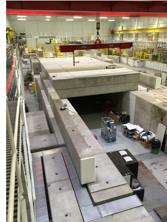
(b) Installation of roof beams
