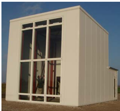
Figure 1. South (DSF) façade of the test facility.
