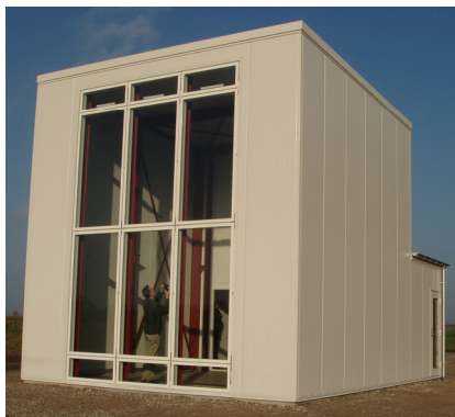
Figure 1. South (DSF) façade of the test facility.
