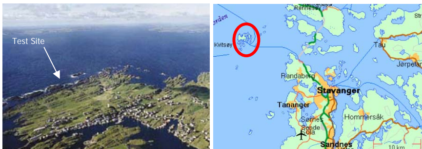
Figure 2. Photo montage and location of pilot plant to be installed on the west coast at the island of Kvitsøy, near Stavanger, Norway, courtesy of WaveEnergy AS.
