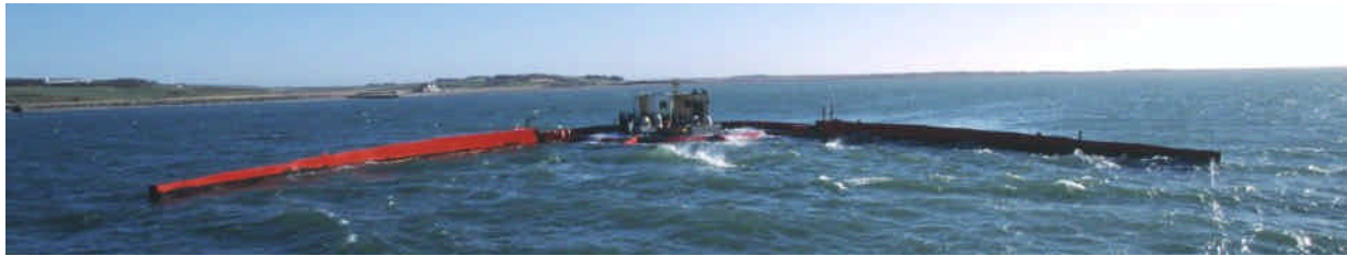
Figure 3: Wave Dragon prototype. Approaching waves are concentrated by the reflector towards the ramp.
