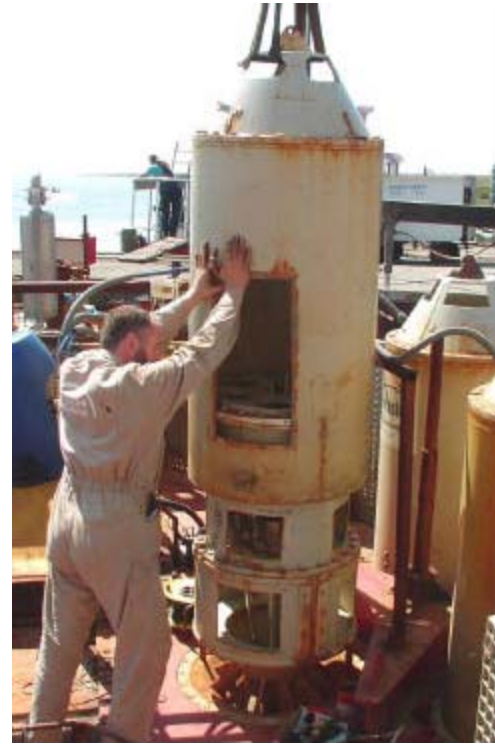
Figure 11: Reinstallation of turbine.
