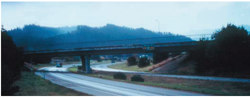
Figure 1. North side view of Painter Street Overpass.
