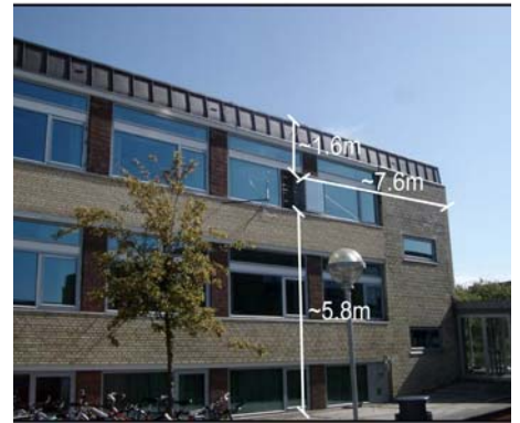
Figure 4.20. Position of the opening in the wall.
