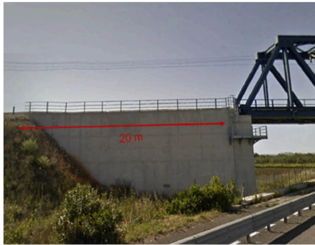
a.1 Wing walls
