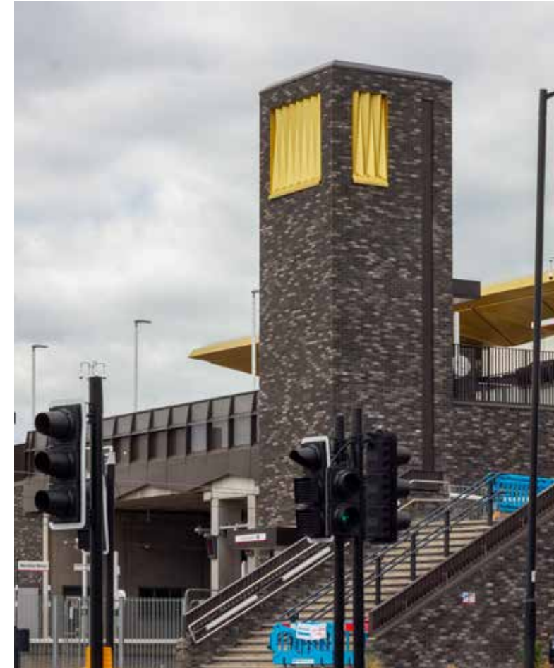
Meridian Water Station
