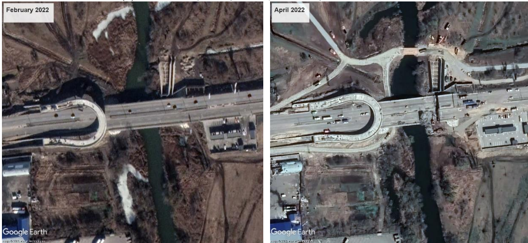
(d) B17: LoK H ; DL M ; CCD GL =0.351; CCD LOC =0.521 (on the right a temporary diversion route was constructed to bypass the bridge)
