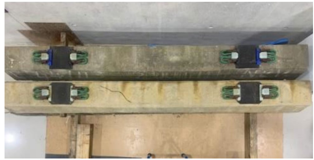
a) Inclined cracks
