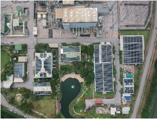
Fig. 5. GTCC power plant 700 MW which installed 980 kW solar PV.
