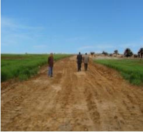
a) High Plasticity Subgrade
