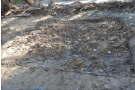
(a) The hole at rainy condition (3-2-2011)
