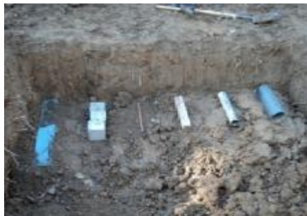
(c) Third layer at depth 0.45 m
