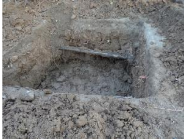
Figure (5) The early stage of the excavated hole.
