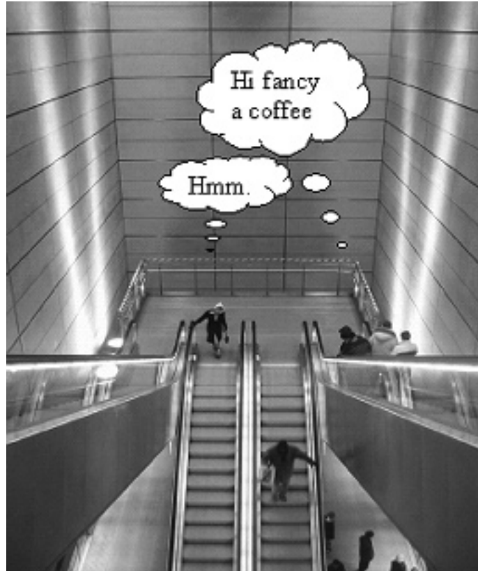
Figure 11. Escalator at the Copenhagen Metro
