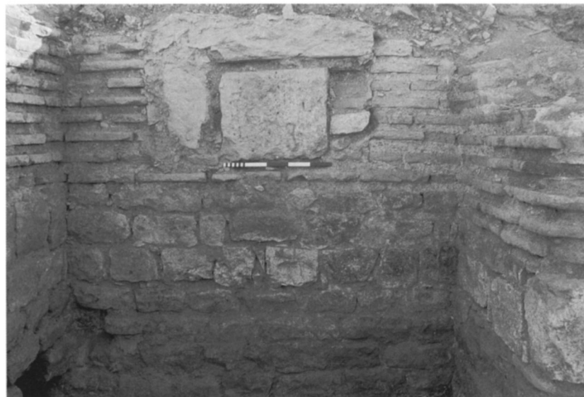
8 Trench XC, Structure 1, northeastern wall (W137) of vaulted room; drain at north corner, shown bottom left (neg. AM01/07/36A)
