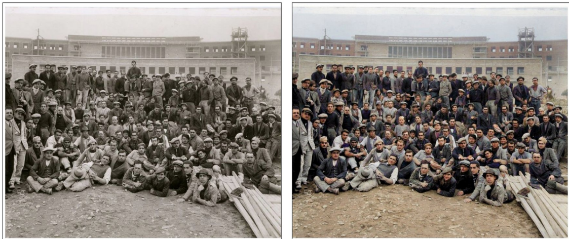
1938/39, the CMC Ravenna construction team pose in front of the majestic almost completed Colonia Varese.
