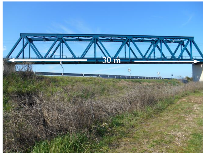
Figure 6. Metallic railway bridge across a motorway (San Severo, Italy).
