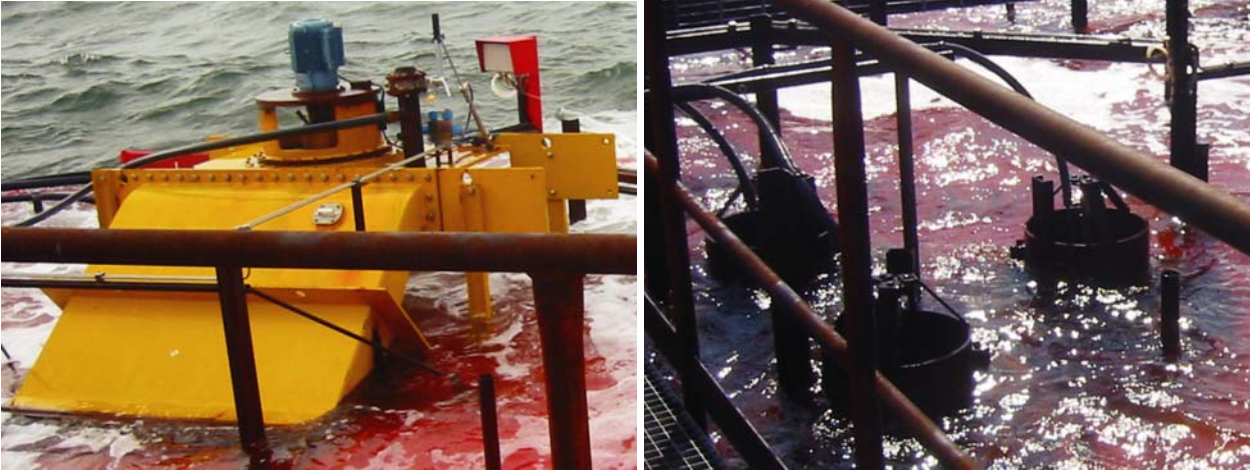
Figure 4. Left: The siphon turbine on board the prototype in Nissum Bredning. Right: The dummy turbines on board of the prototype in Nissum Bredning.
