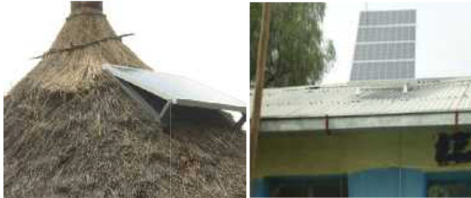
Figure 2: Mounted solar panels in the thatched and metal roofs of the rural houses [18]
