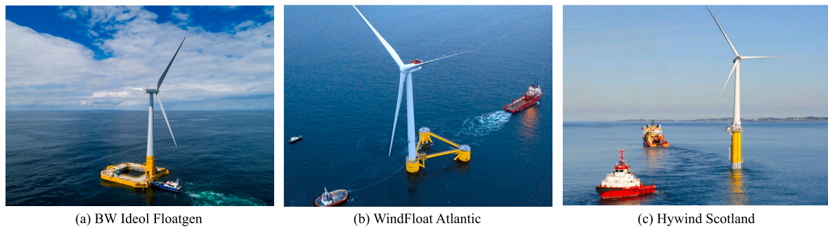
Fig. 4. Examples of barge, semi-submersible and spar foundation specific designs and project towing operations: (a) BW Ideol Floatgen, (b) WindFloat Atlantic and (c) Hywind Scotland projects.
