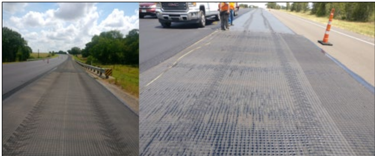
Figure 3: Installation of Geosynthetic Reinforcement in Test Sections
