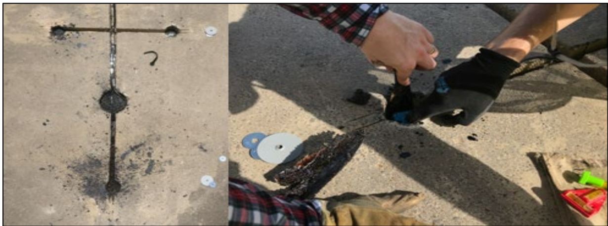
Figure 6: Geophone Installation in HMA
