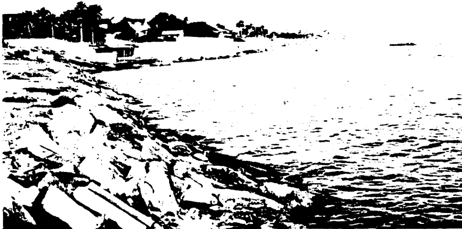
Figure 12. Concrete riprap used as shoreline protection near Ward Island, southern Corpus Christi Bay.
