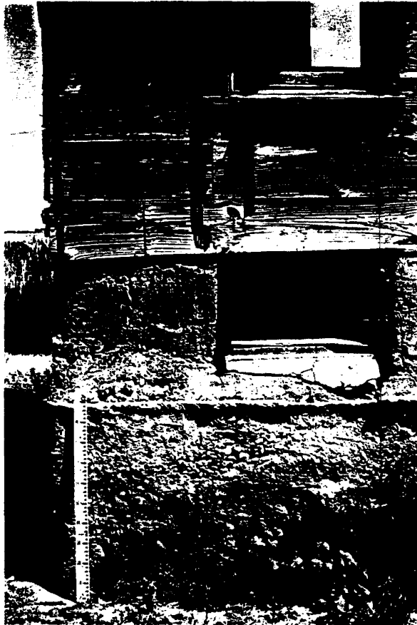
(B) Detail of exposed foundation, the lower half of which retains impressions of trowel marks and root traces. The concrete forming this part of the foundation was poured against the wall of a shallow excavation. The original ground level is indicated by the rim of concrete at the top of the one-meter scale bar.
