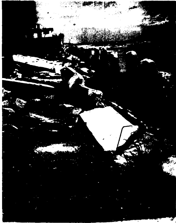
Figure 8. Remnants of a reinforced concrete bulkhead destroyed by Hurricane Alicia, Sea Isle subdivision.
