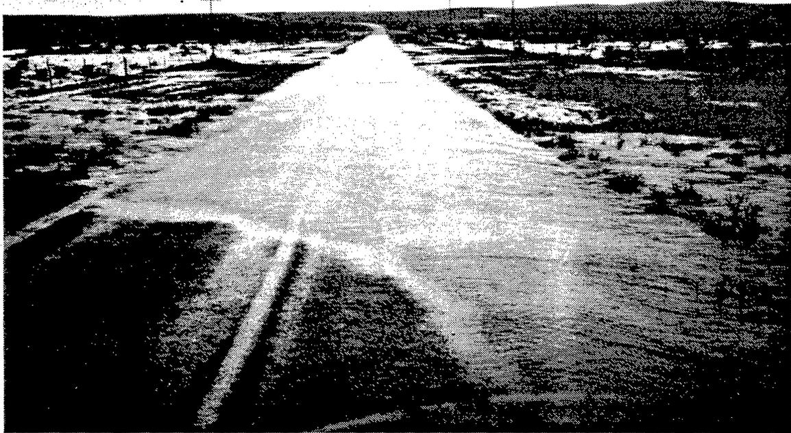
Figure 43. Photograph of flooding at Antelope Draw where it crosses Ranch-to-Market Road 1111. The flood created a body of water 2 ft (0.6 m) deep and as much as 200 to 300 ft (60 to 91 m) across. Duration of flooding was very brief, and the highway became passable almost as soon as rainfall terminated.
