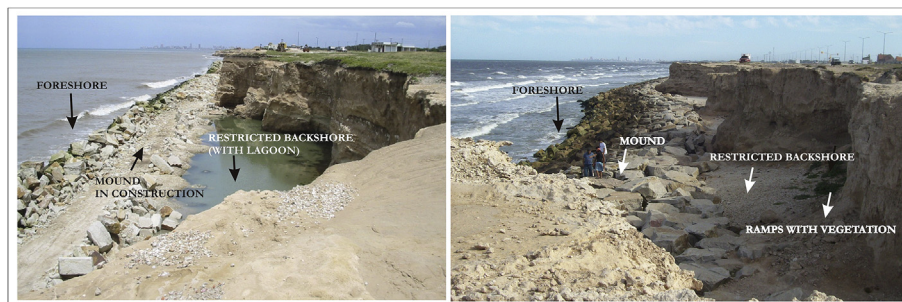
Fig. 7. Comparative photographs in Santa Helena coast during (2011, on the left) and after the mound construction (2013, on the right). It can be seen the temporary ponds in the restricted backshore during high tides or surge storms, and the ramps with vegetation during low tides.
