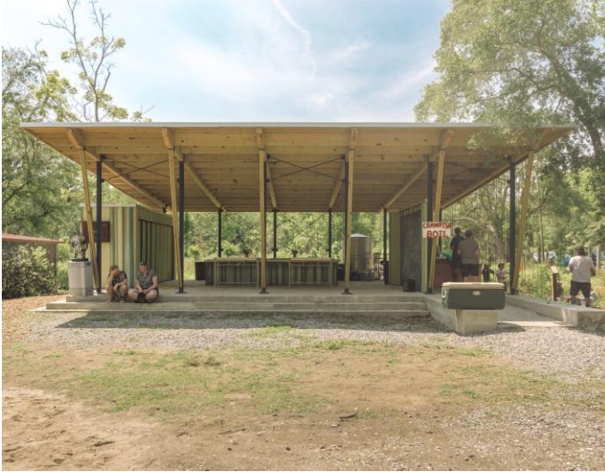
Figure3: The final result of the outdoor teaching space at Sugar Roots Farm (Small Center).
