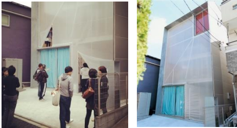
Figures 7,8: House idiosyncratic view with 3m set back, two asymmetrical window positions, two unzipped openings at front façade polymer membrane and gathering atmosphere at private / public house front area; [Moroney, 2012]
