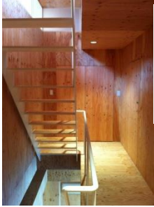
Figure 21: First floor plywood covered level with three room nr.3,4 and 5 and toilet entrances; [Hirano, 2012]
