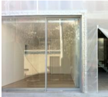
Figure 18: Full height glazed north wall of room nr.1 with two-slide opening to front part of house lot; [Hirano, 2012]
