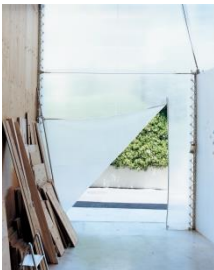
Figure 9: Unzipped membrane entrance and doma area with continuation of outer concrete floor to interior flooring; [Hirano, 2012]
