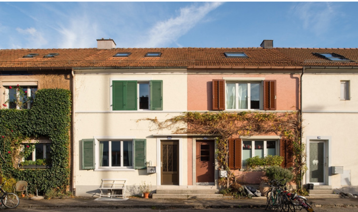
Bernoullihäuser, cooperative single-family homes, Zurich, 1929 (© photo: Julie Haller, 2015, Baugeschichtliches Archiv/City of Zurich)
