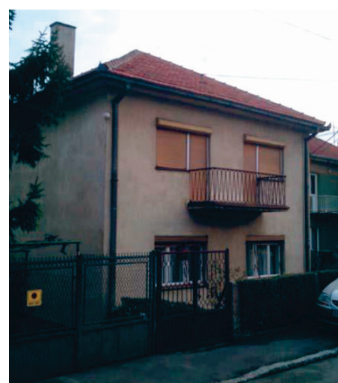
Figure 2. Typical free-standing house from 1946 to 1970 [25]
