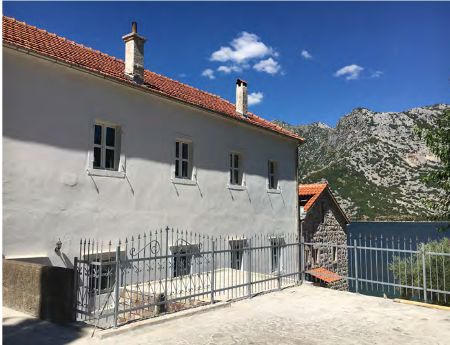
Figure 7. The northern façade of the new monastic quarters (Photo: M. D. Petrović, 2019)
