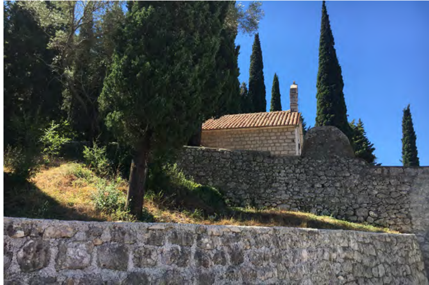
Figure 2. The Church of Saint George, western façade (Photo: M. D. Petrović, 2019)
