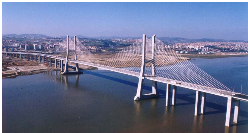
Fig. 1 – Cable-stayed component of Vasco da Gama Bridge
