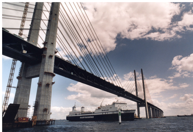
Fig. 23: Ship passing the bridge during construction
