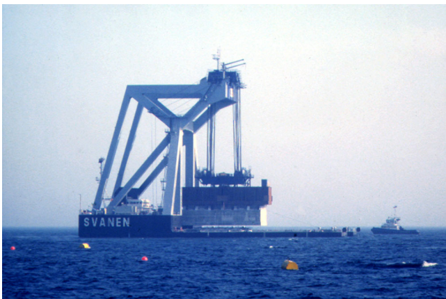
Fig. 5: Placing a caisson by Svanen
