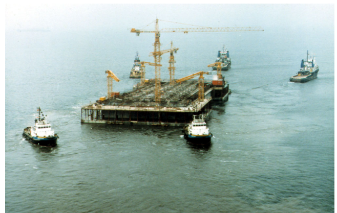
Fig. 9: Placing of anchor block caissons
