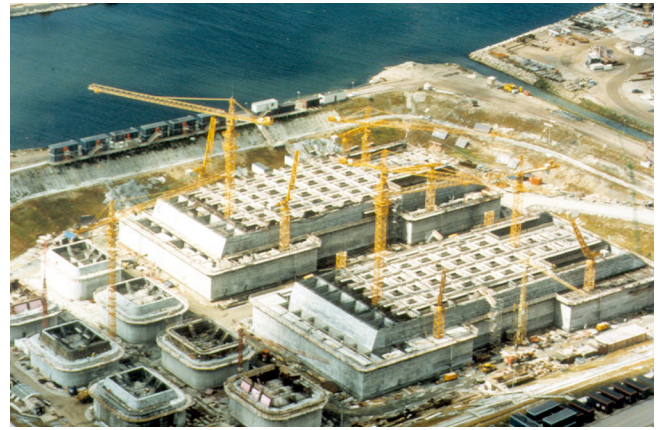
Fig. 8: Anchor block caissons in dry dock
