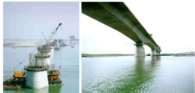
Fig. 31: Casting of pile caps and completed bridge
