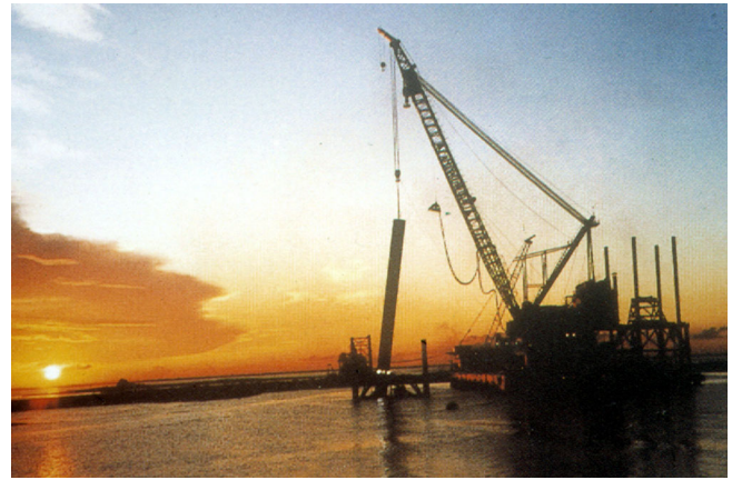
Fig. 30: Driving a 3.15 m diameter pile
