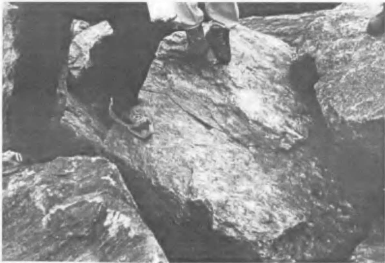
Photo from Norwegian berm breakwater
